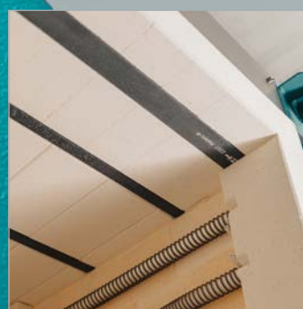
Special ROHDE ceiling construction prevents cracking and thus unwanted contamination
