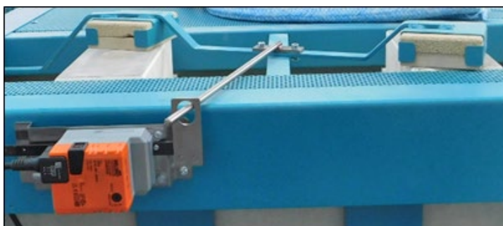
Figure 25: Automatic exhaust air flap
